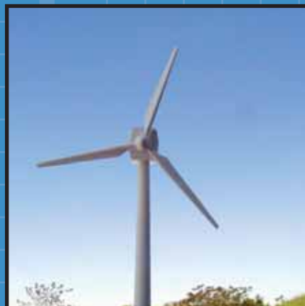
Wind Turbine Electricity
